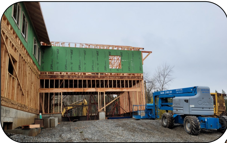
This is a view of the garage of the new convent.
