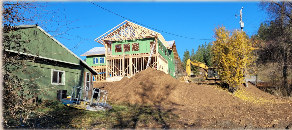
Work progresses on our new convent.
