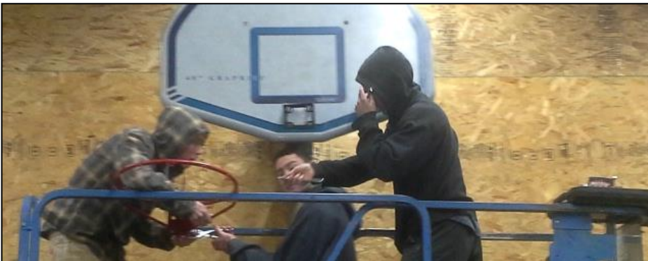
We helped Frater Anthony install a new backboard in the gym.
