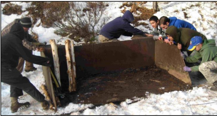
This job was a lot harder than it looks!
