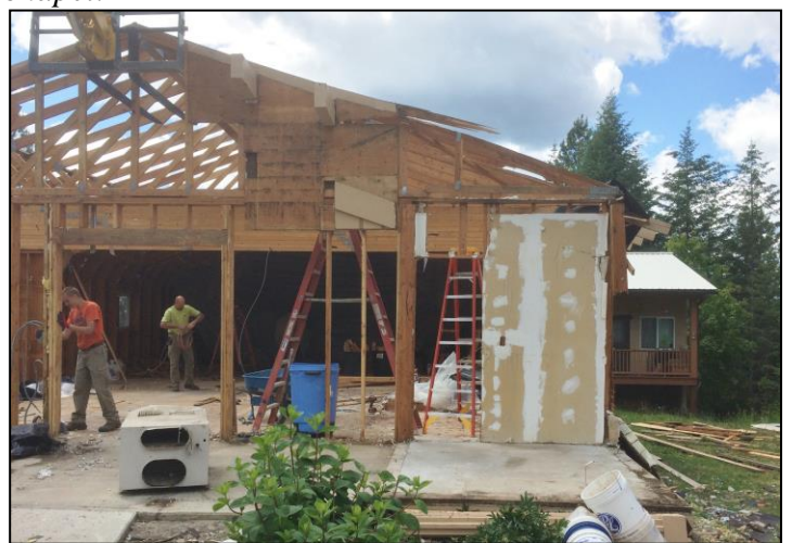
The entire front of the church has been removed, as part of the remodel project.
