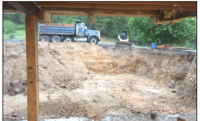
The hole is dug to prepare to extend the church basement.
