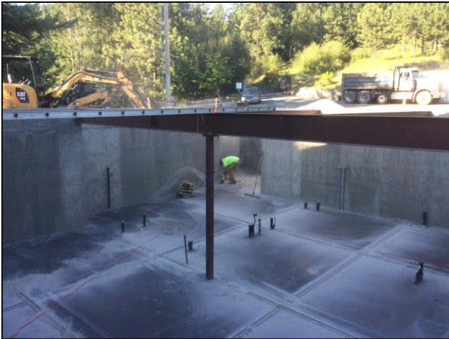
View of the new basement extension after the concrete is poured.
